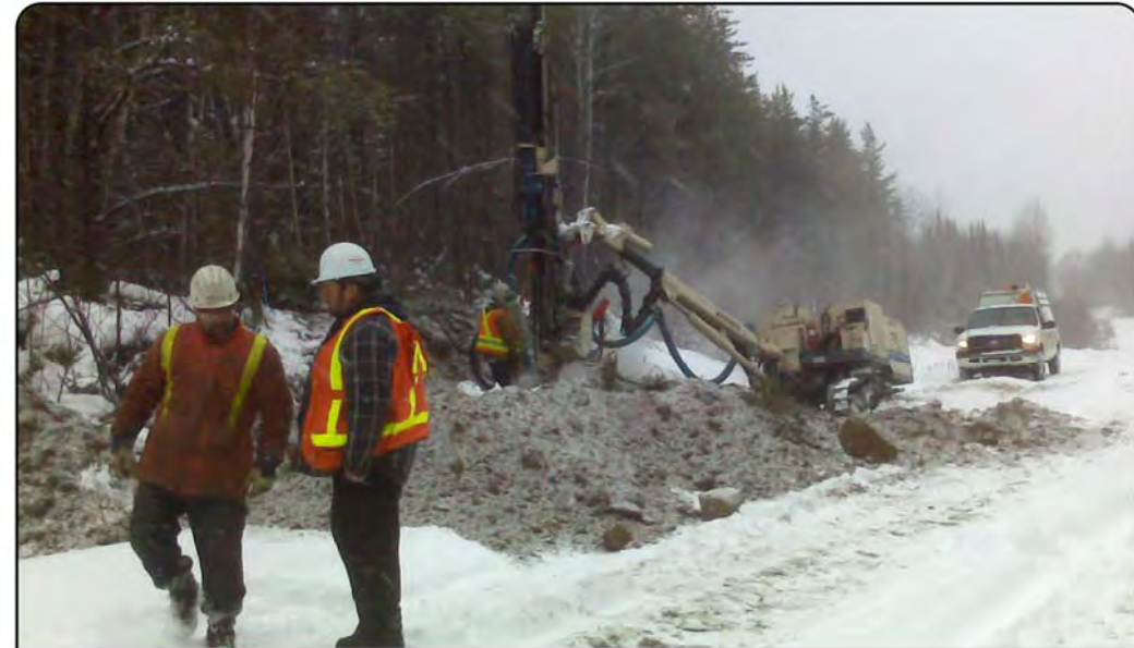
Drilling Operation Supervision
