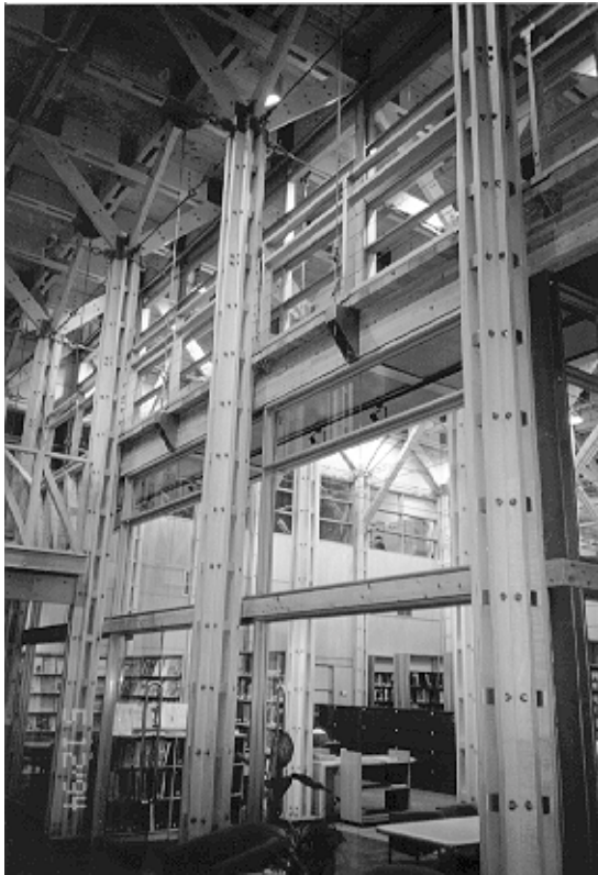
Figure 1. Tembec's laminated veneer lumber used as support structures in Forintek Canada's new laboratory and research centre in Québec City, Québec.
