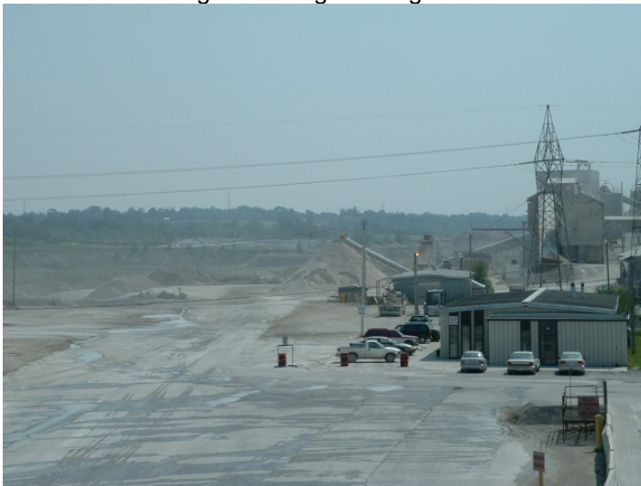
Figure 4: Large un-vegetated surfaces
